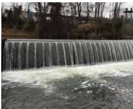
Lindsey Bridge Dam before retrofitting
