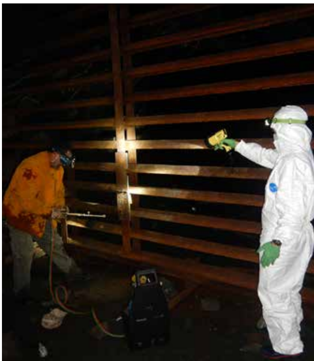
Conservation Technician, Joe Tomcho, prepares to fix an interior gate while Wildlife Diversity Technician, Kristi Confortin, provides a light source.
