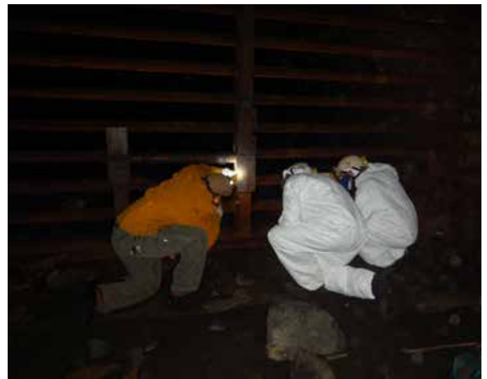
Conservation Technician, Joe Tomcho, Western Wildlife Diversity Supervisor, Kendrick Weeks, and Wildlife Diversity Technician, Kyle Shute, repair the bat gate inside an Avery County mine. (Katherine Etchison)
