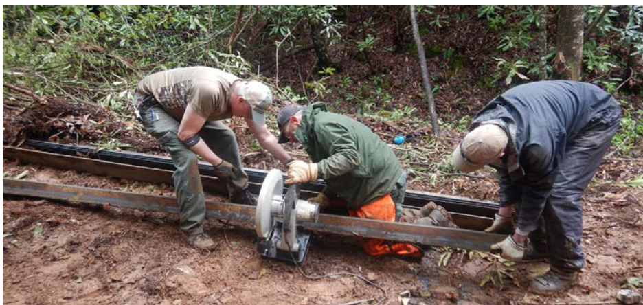
Nantahala National Forest Wildlife Biologist, Johnny Wills, Conservation Technician, Brandon Allen, and Franklin Depot Team Leader, Mike Parks, prepare to cut steel for a mine gate. (Katherine Etchison)
