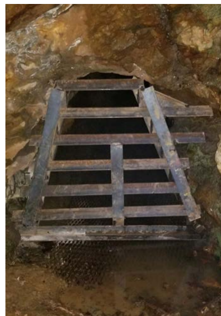
A Macon County mine entrance on the Nantahala National Forest after gate installation (Johnny Wills/USFS)
