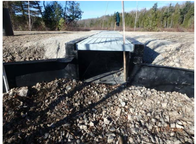
Figure 2. Examples of wildlife exclusion fencing used to reduce bog turtle mortality on roads (from Animexfencing.com ). This type of fencing will be installed using PFW funds at a property in North Carolina to direct bog turtles and other small wildlife into existing under-road passages. (Gabrielle Graeter)
