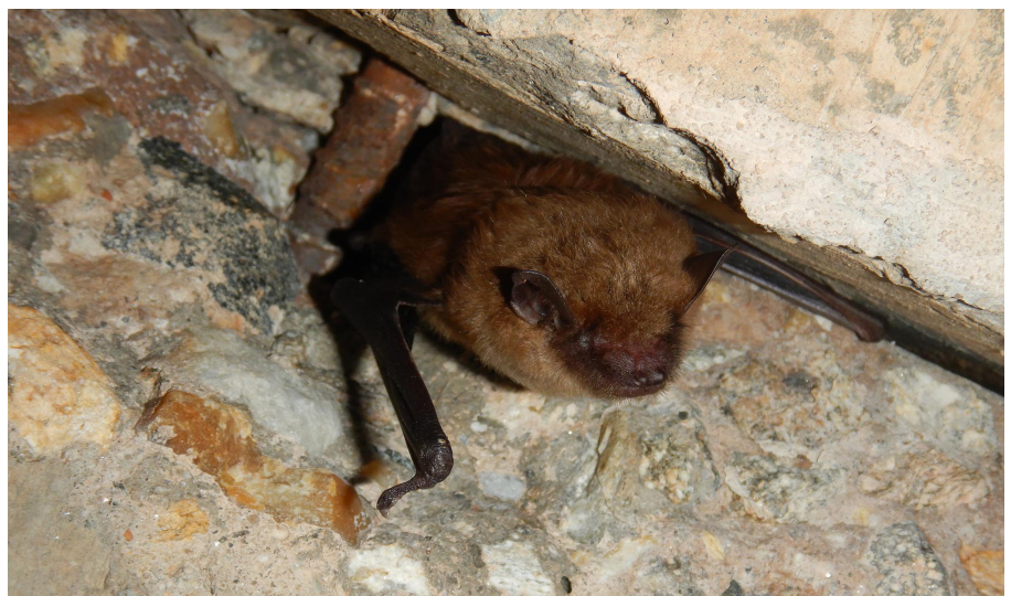
A hibernating big brown bat in a McDowell County culvert. (Katherine Etchison)
