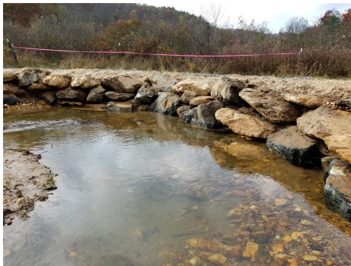
Figure 2. Large boulders and matting were used to stabilize the formerly eroding stream bank. The bog edge is immediately behind the pink flagging. Large gravel was laid down adjacent to the boulders to ensure the farmer could access his hayfield again. (Photo: Gabrielle Graeter/NCWRC)
