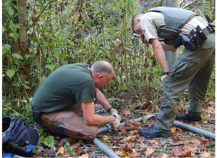
Western Wildlife Diversity Supervisor, Kendrick Weeks, and Senior Officer, Jared Thompson, install hinges to a recently breached gate.
