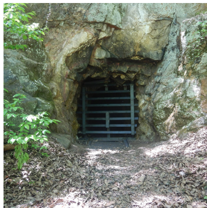
Entrance to a mine on Crowder's Mountain State Park before and after gate installation (Photos by Katherine Etchison)
