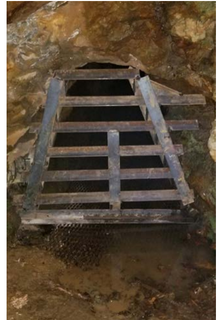
A Macon County mine entrance on the Nantahala National Forest after gate installation (Johnny Wills/USFS)
