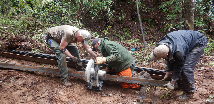
Nantahala National Forest Wildlife Biologist, Johnny Wills, Conservation Technician, Brandon Allen, and Franklin Depot Team Leader, Mike Parks, prepare to cut steel for a mine gate. (Katherine Etchison)
