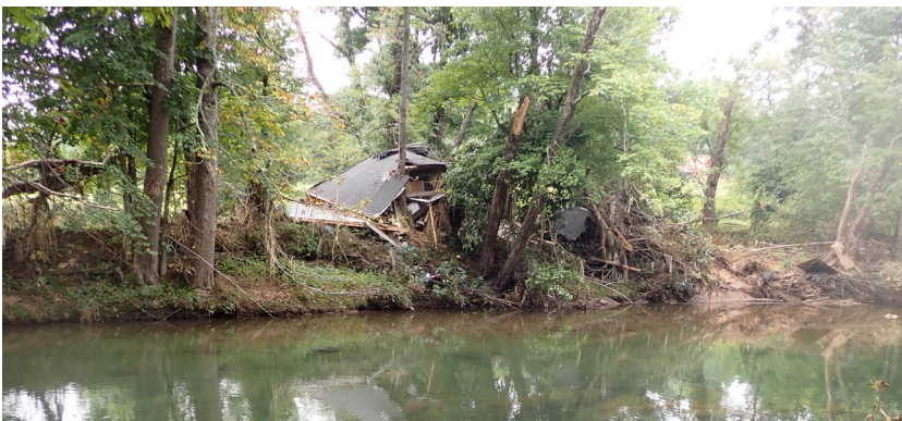
Flooding damage on the East Fork Pigeon River in Haywood County (Dr. Luke Etchison)
