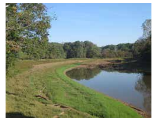
Dewatered impoundment behind Hoosier Dam in fall 2017. Treeline indicates former water level. Exposed banks have been seeded for stability. (Photo NCWRC)
