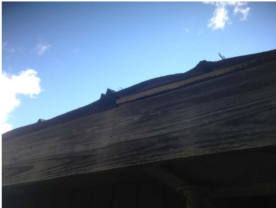
8. Buckled Roofing
