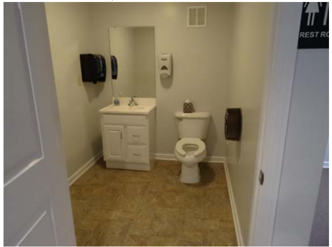
2 nd floor restroom
