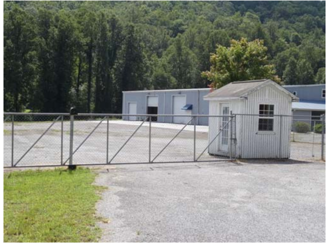
Gate to Paved Lot
