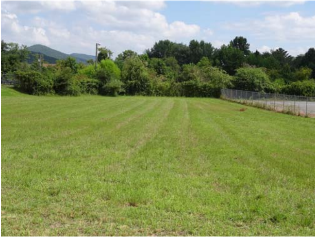
Lot w/ 6" layer of gravel base
