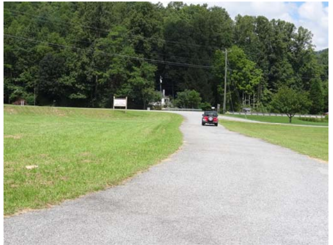
Paved Driveway (North)
