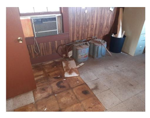
• Photo 3: Rotting floor under ceiling leak
