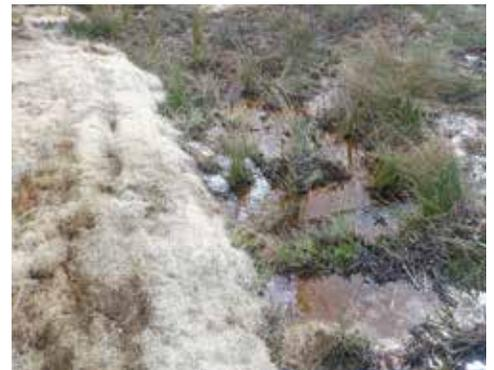
*A close-up view of the stabilized primary head-cut channel, immediately post-restoration, with the log sills in place, erosion matting, and transplanted wetland plants between log sills.*
