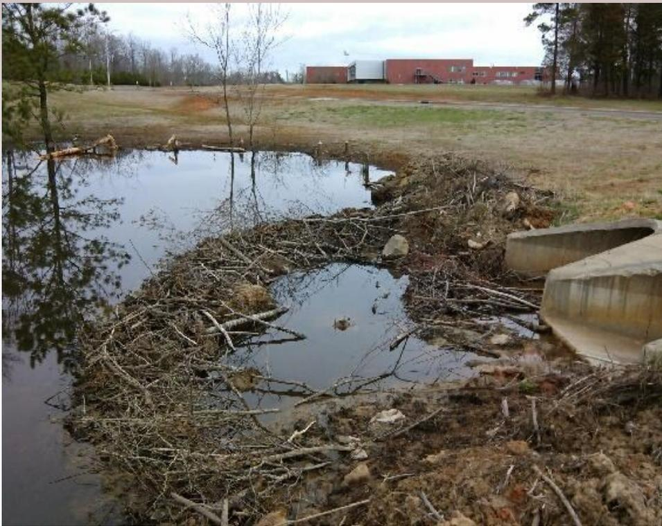
**Before:** A dammed culvert raised concerns for potential flooding at the entrance road to Granville County Central High School near Stem. It was also flooding an adjacent landowner's timber. Photo credit: Todd Menke, USDA Wildlife Services.
