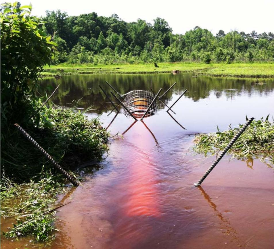
**Left:** Clemson Beaver Pond Leveler, a non-lethal method installed in Franklin County, as a water control device to mitigate damages caused by beaver. Beaver do create excellent wetland habitats and for this landholder, an avid waterfowl hunter, he wanted to try to co-exist with the beaver. Photo credit: Todd Menke, USDA Wildlife Services.
